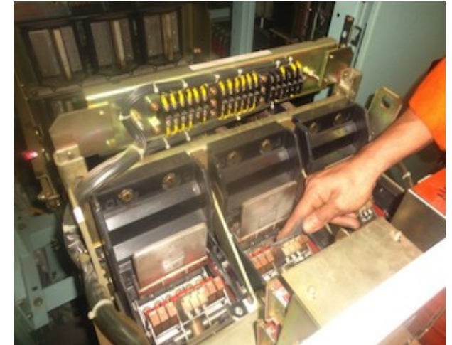
Open Air Circuit Breaker in MSB
